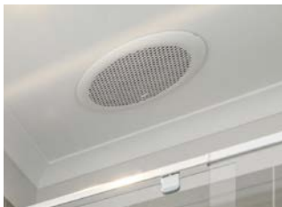
8 Ceiling exhaust fans above showers and to any wet areas without external ventilation
