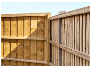
4 Side and rear fencing
