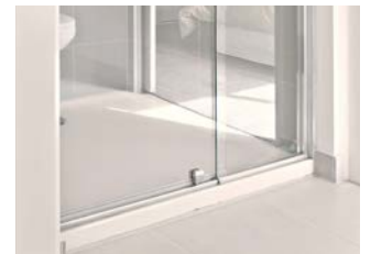
3 Raised tiled shower bases with approx. 1950mm high clear glazed semi-framed shower screen and semi frameless pivot door with silver trims
