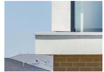
3 Concrete tile or Colorbond corrugated metal roof. Colorbond fascia, gutter and downpipes.
