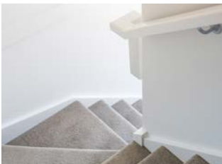
7 Staircase with plaster dwarf wall balustrade with painted shadow line capping, carpeted MDF treads & risers, painted timber wall rail and pine stringers
