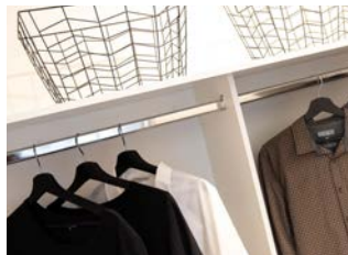
8 Wardrobes with 2100mm high vinyl sliding doors, 1No melamine fixed shelf and 1No chrome hanging rod
